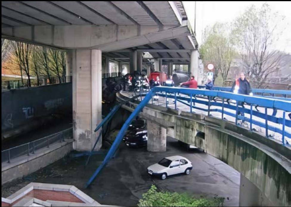
ABOVE: Use of the old style, non-tested, Mailloux parapet design ceased in Belgium following the introduction of the European Standard EN1317.2
